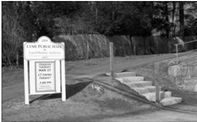
New granite steps were installed in March.
